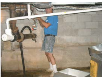
Habitat volunteer Jim Gregg removing copper plumbing to be recycled.
